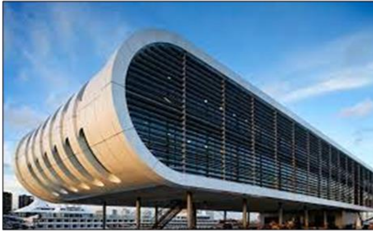
Figure 7. Contemporary Building Design
